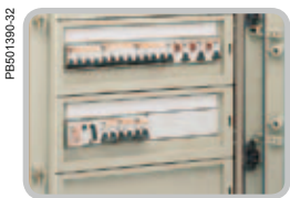
Detail from the circuit-marking system.
